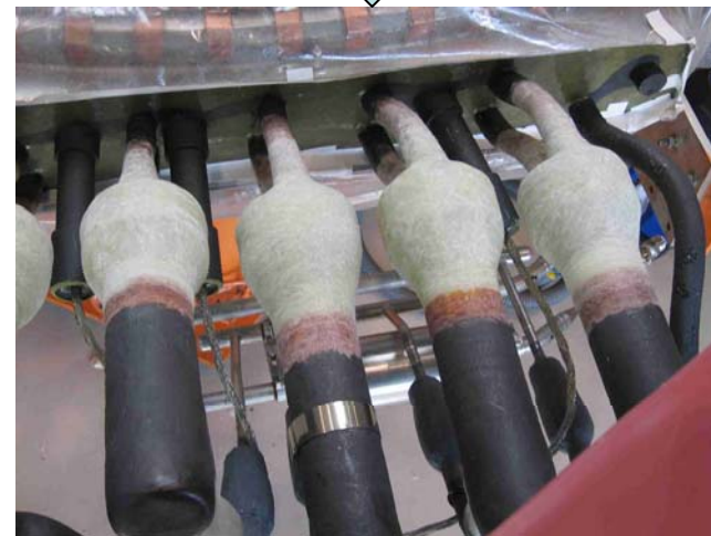
3. Repair of the insulation in the affected region
