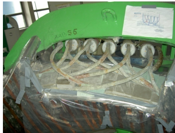
5. Repair of Winding Pack
